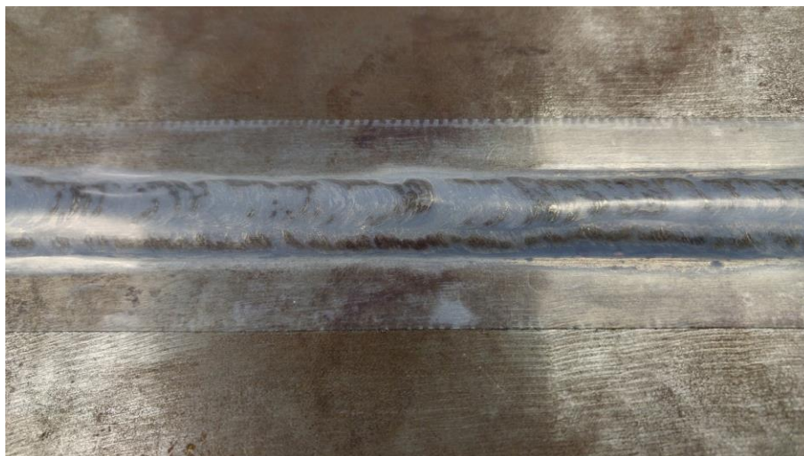
Figure 71. Protective tape applied directly on weld
